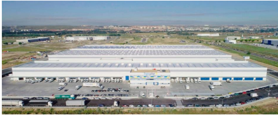
Figure 4- Dispnal's Logistic Centre in Madrid, Spain. Source: (Dispnal, 2024)
