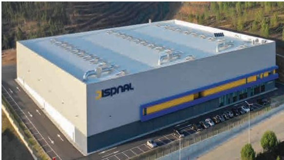
Figure 2- Dispnal's Head Office, Baltar. Source: (Dispnal, 2024)
