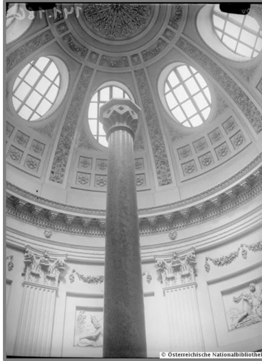
Figure 1: Cupola hall. Look into the vault with a free-standing column. Vienna, 1900
