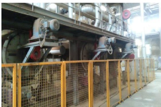
Figure 3.21 Shows the pop chambers present in GMT section 1 it has 3 chambers
