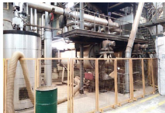
Figure 3.22 Shows the pop chambers present in GMT section 3 it has 2 chambers
