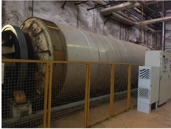
Figure 3.23 Dryer in GMT section 1
