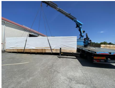
Figure 45 - Example of handling the pallet.
