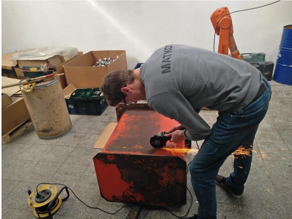
Figure 34: Cutting the pedestal along the first line
