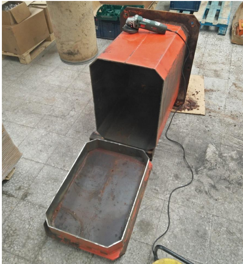
Figure 36: Pedestal top plate cut off
