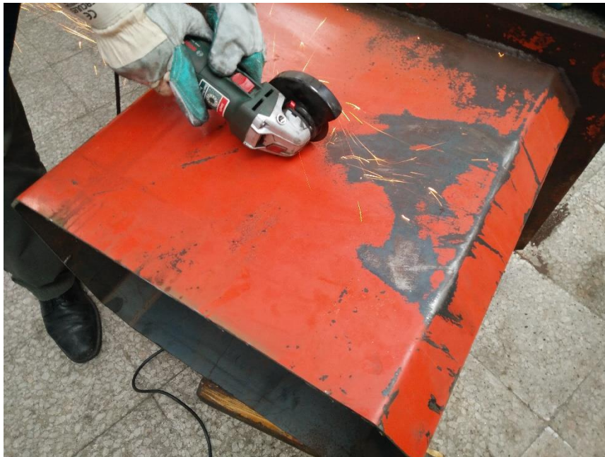
Figure 37: Cutting the pedestal along the second line
