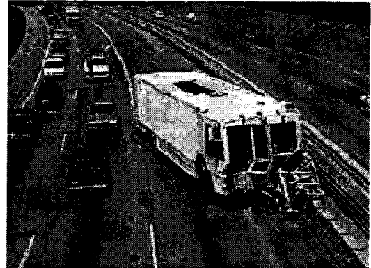
Fig. 4 - Moving the concrete jersey barriers dividing the highway [17]
