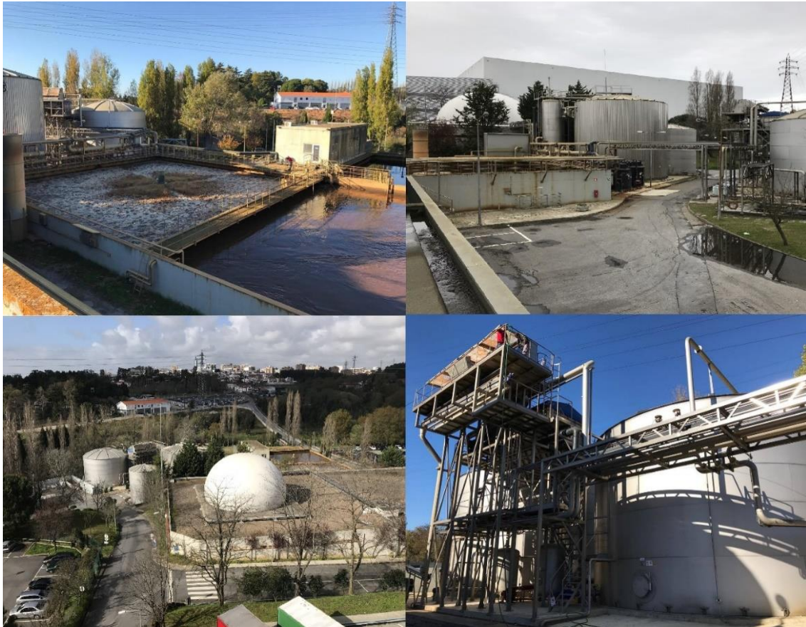
Figure 33 - Clockwise: Aerobic Treatment; Anaerobic Treatment; Pre-Treatment; Overview of the WWTP
