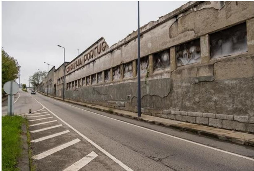
Figure 28- Façade of the now demolished Companhia Portuguesa do Cobre
