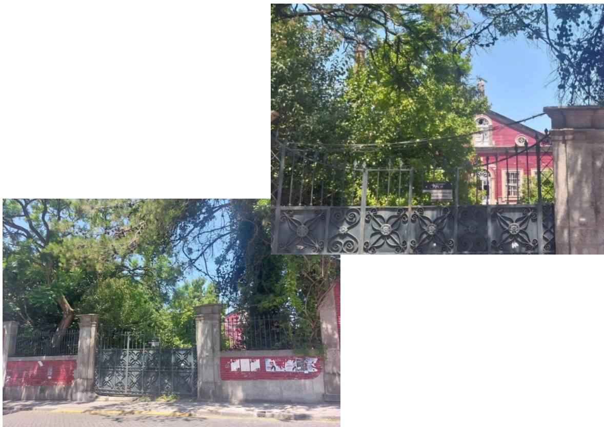
Figures 54 and 55- Gate and elements of the interior of the building
