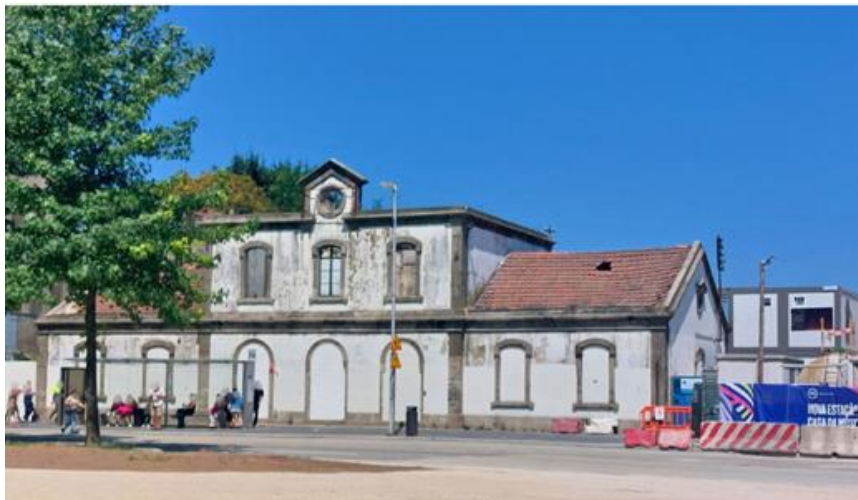
Figure 47- Façade of the station
