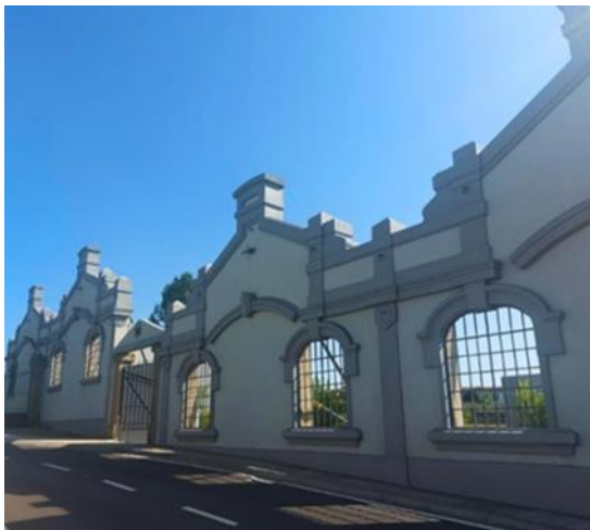
Figure 14- Façade of the Building Preserved (another perspective)
