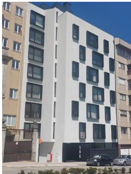
Figure 9- Residential Building Constructed
