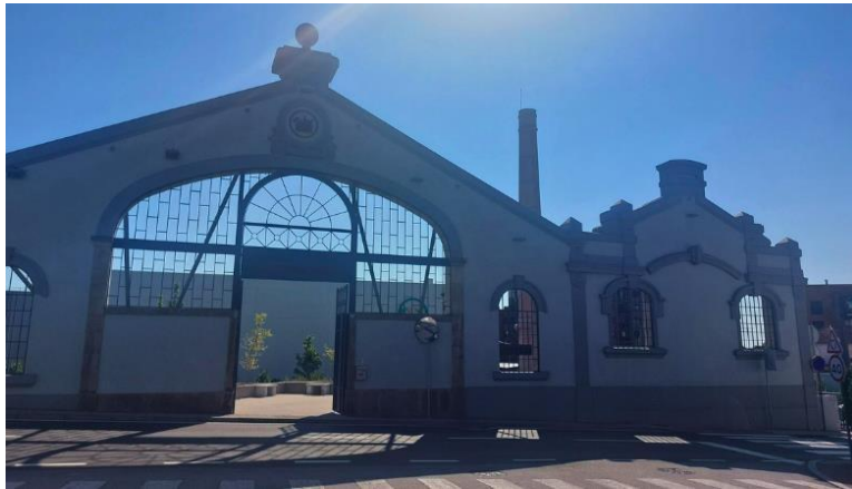
Figure 13- Façade of the Building Preserved (Photograph taken by the author, August 2024)
