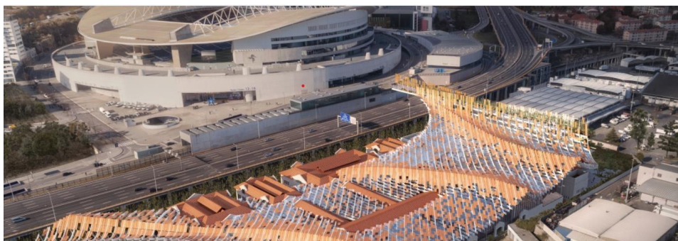
Figure 36- Overall look of the project in the space
