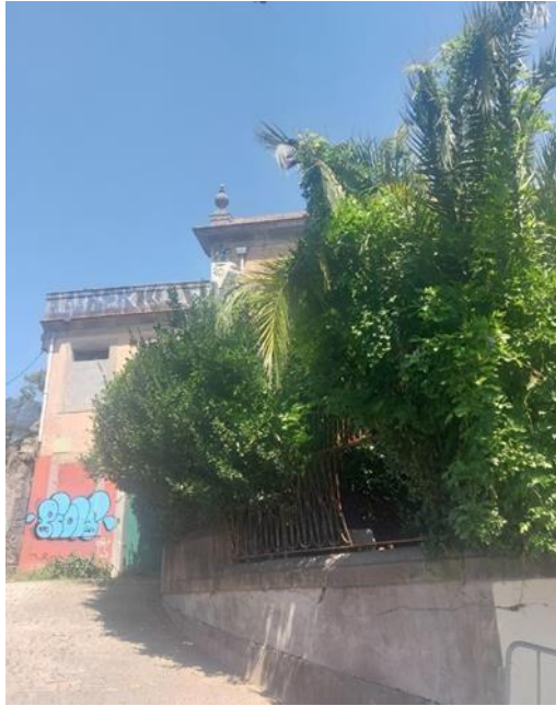
Figure 59- Showcasing the vandalism and invasion of the space
