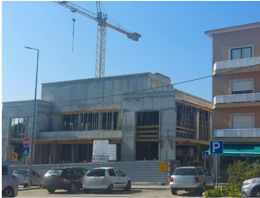
Figure 42- Construction status of “Oficina Municipal das Artes”
