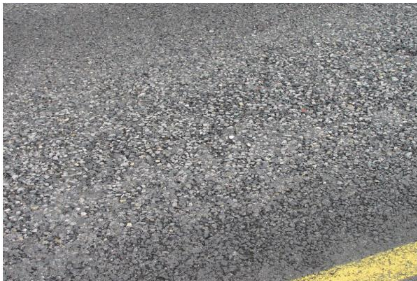
Figura 25: Desgaste (WSDOT, 2020)
