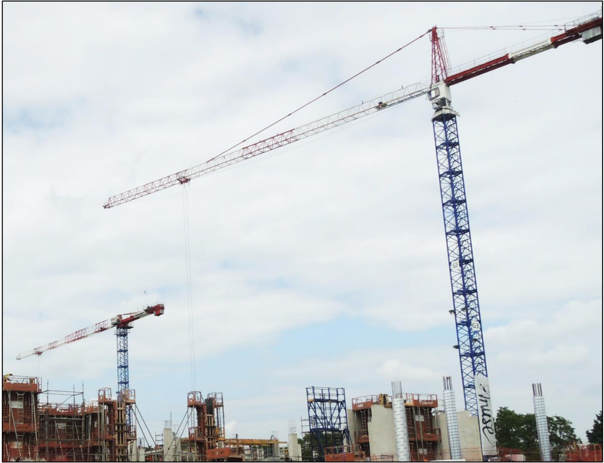
Figure 2.10 – A high-top crane (front) and a flat-top crane (back) (Project Muse, Metz, France)
