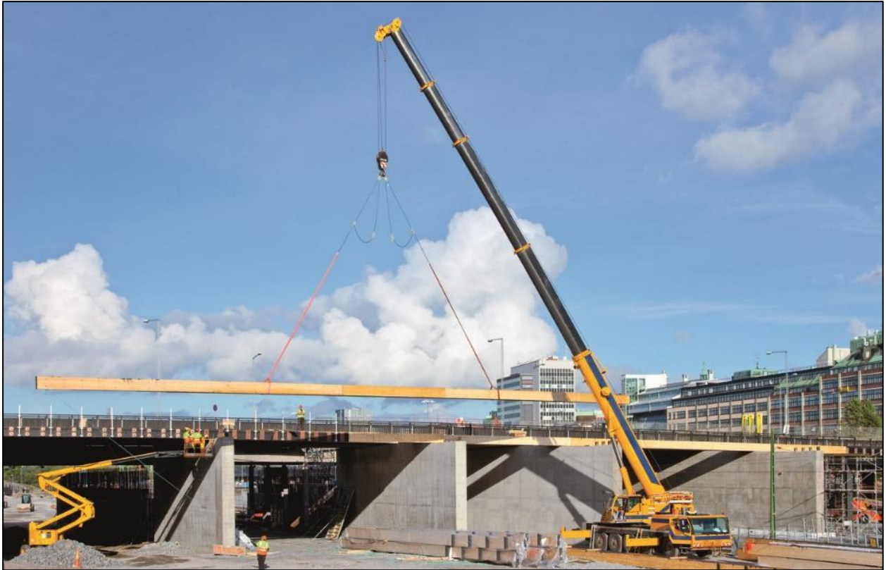
Figure 2.8 – A mobile crane on a construction site
