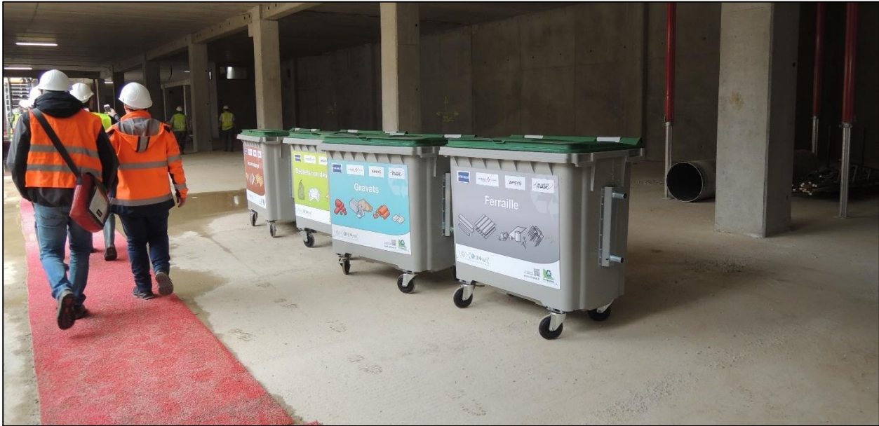
Figure 4.38 – Site visit in Metz; red carpet indicating workers' pathway; recycling point
