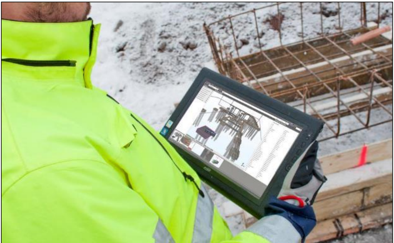
Figure 2.4 – BIM use on construction site, using Tekla’s BIMsight app on a tablet ( https://goo.gl/J0aIPZ )
