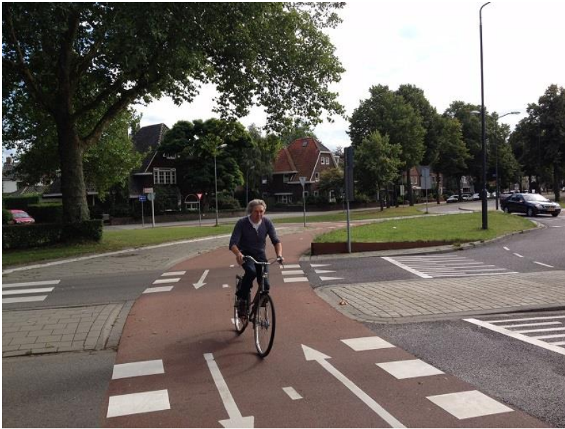
Figure 4- An example of the integration of bicycle infrastructure within Dutch road traffic. The red paths on the floor represent the bicycle lanes. Source: (Andersen, 2019)
