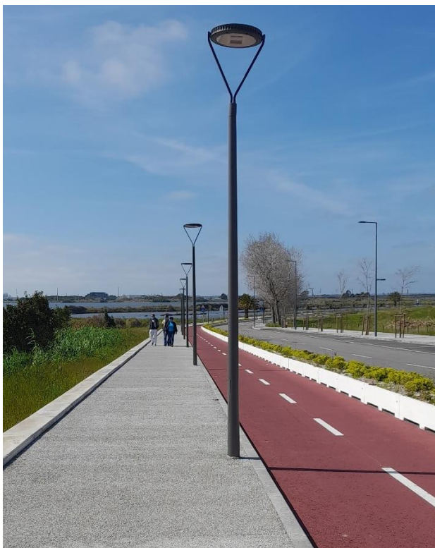
Figure 8- This image of Rua da Pega, in Aveiro represents the road model that provides sufficient safety to cyclists and pedestrians, by creating a physical barrier between these and motor vehicles. Source: Author
