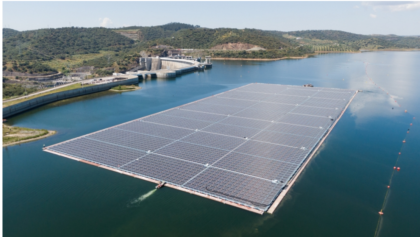
Figure 1.1: The floating PV solar plant in the Alqueva Dam, the largest on a reservoir in Europe.
