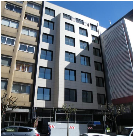
a) Fachada principal
