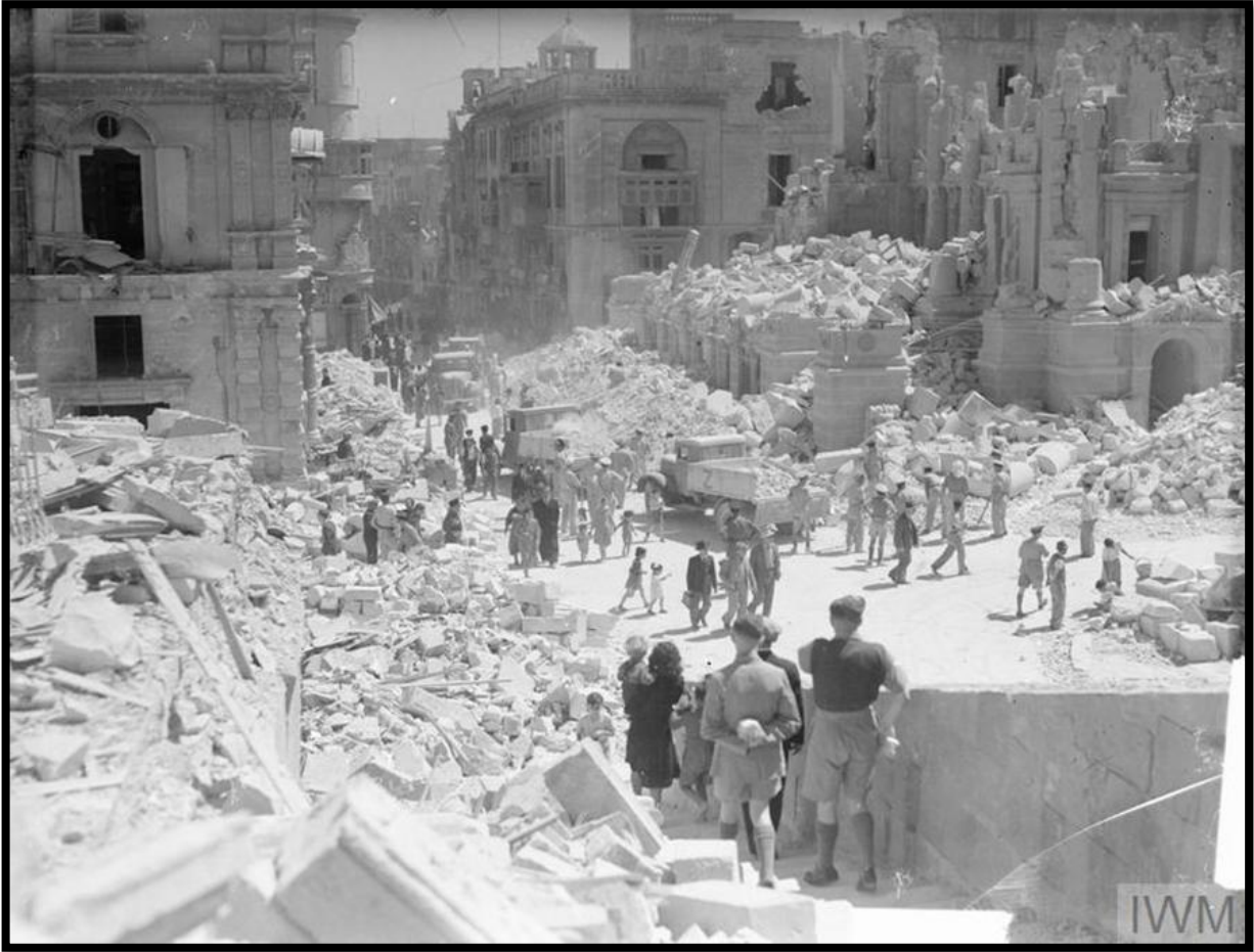
Fig. 433 A heavily bomb-damaged street in Valletta, Malta. This street is Kingsway, the principle street in Valletta. Service personnel and civilians are present clearing up the debris.
