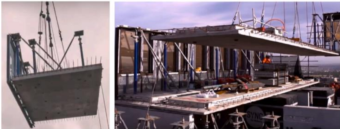
Figure 4 - Example of Modular construction process in site.
