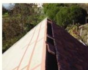
Fig. 43 – Remate com fita Ondufilm
