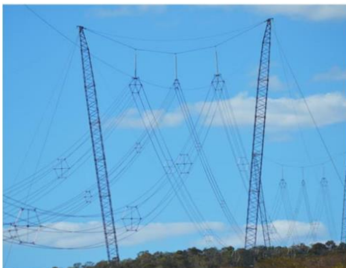
Figura 9 - Torre Cross Rope [29]
