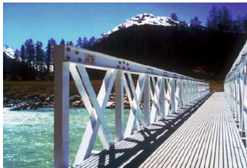
Figure 2.1 - Pontresina footbridge in Stwizerland
