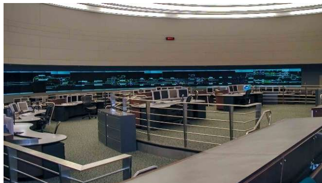
Figure 2.10: ATS System. (Railworks, 2024)
