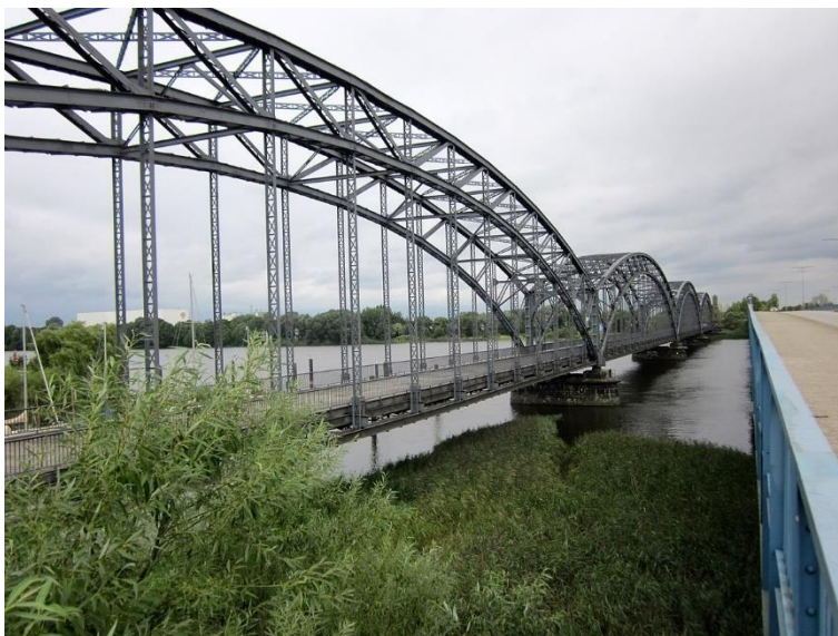
Figura 2.6 – Ponte Harburger Elbbrücke (pedonal)
