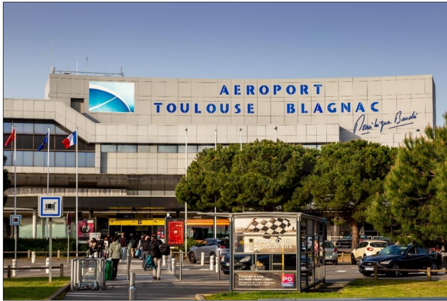
Figure 12 - Toulouse-Blagnac Airport (TLS) (Source: v1 Images: Aviation Media)
