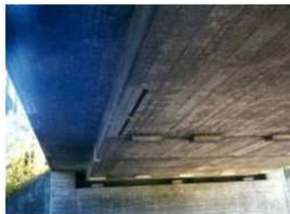
Figure 2.9 – Bridge strengthening with FRP (Ibach bridge, 1991, Switzerland) (Cress, 2000)
