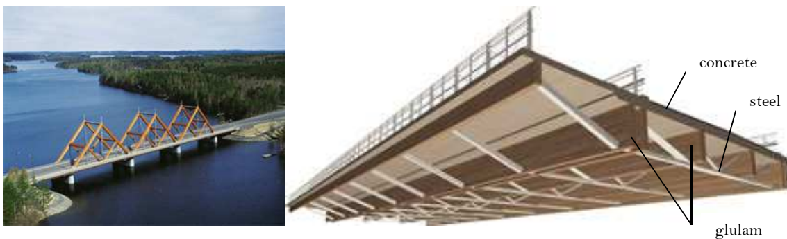
Figure 2.16 – Vihantasalmi bridge, Finland
