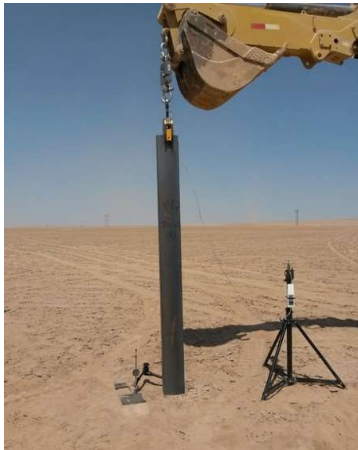
Figure 31 - Ramming and Pull-out Test
