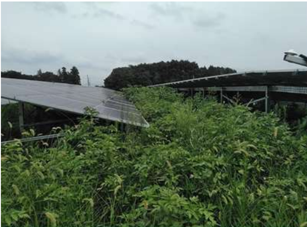
Figure 57 - High grass covering lower modules.
