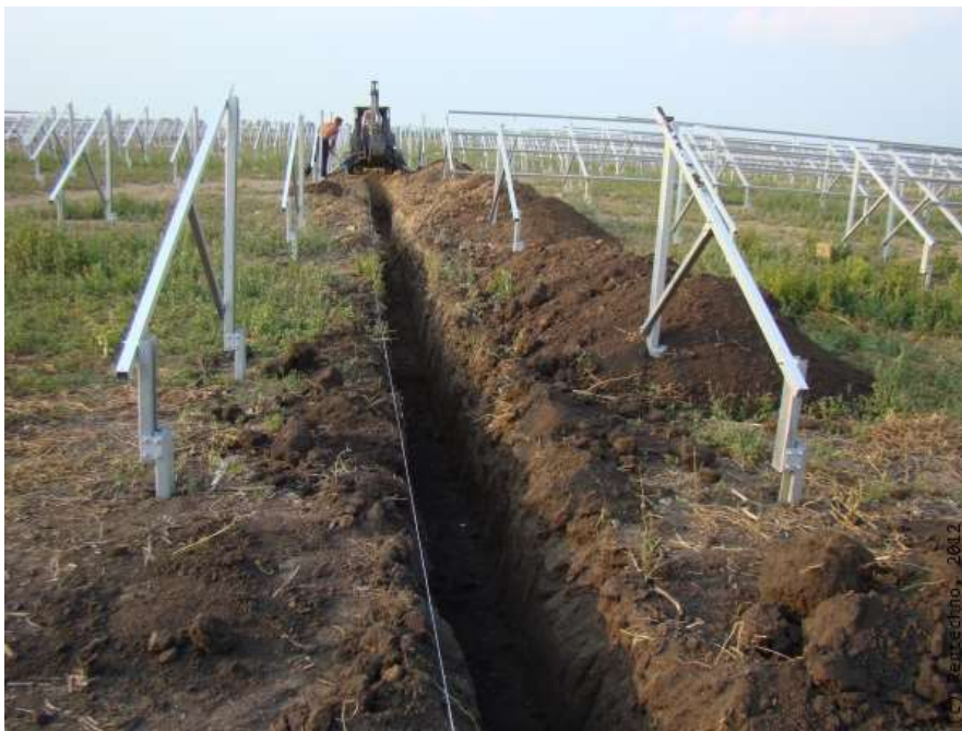
Figure 44 - Trench for cables being dug between the modules mounting structures.
