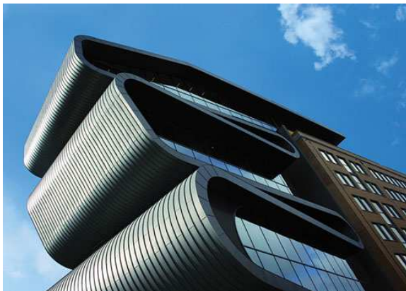
a) Unicore Office Building, Bélgica
