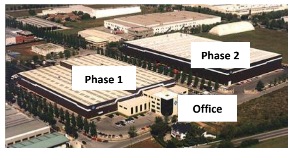
Figure 7 - Gestamp Palau S.A. facilities
