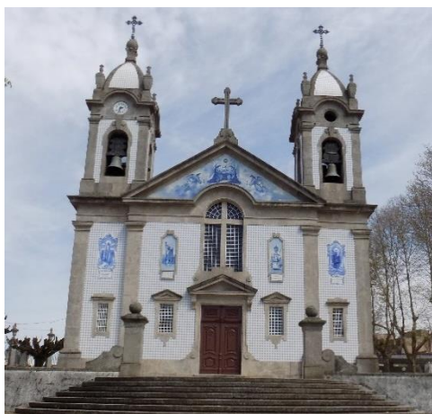
a) Fachada Principal
