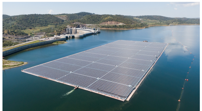
Fig. 1: The floating PV solar plant at the Alqueva reservoir.
