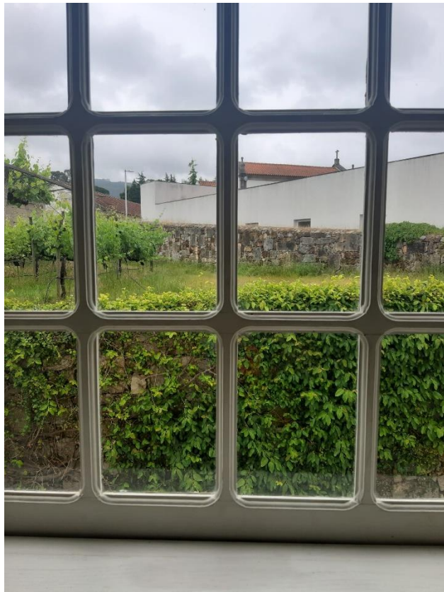
Figure 44: MIEC view from inside, 2021
