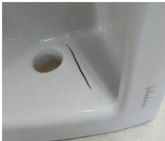
Figure 18 – Cracks in sanitary ware
