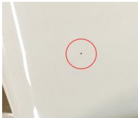
Figure 20 – Stains in sanitary ware [47]
