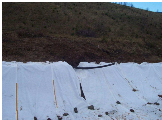
Figure 1.21: RAPS pond covered with plastic foil.
