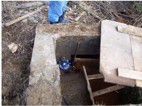
Figure 1.20: Constructed wetland input (P3C)
