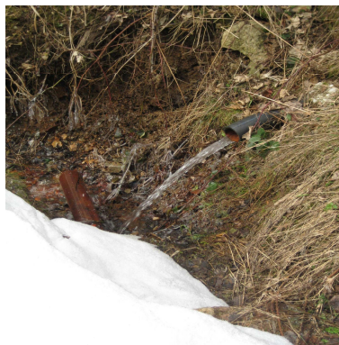
Figure 1.26: Constructed wetland output.
