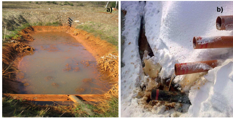
Figure 1.24: a) Sedimentation pond. b) Set of four drainage pipes.
