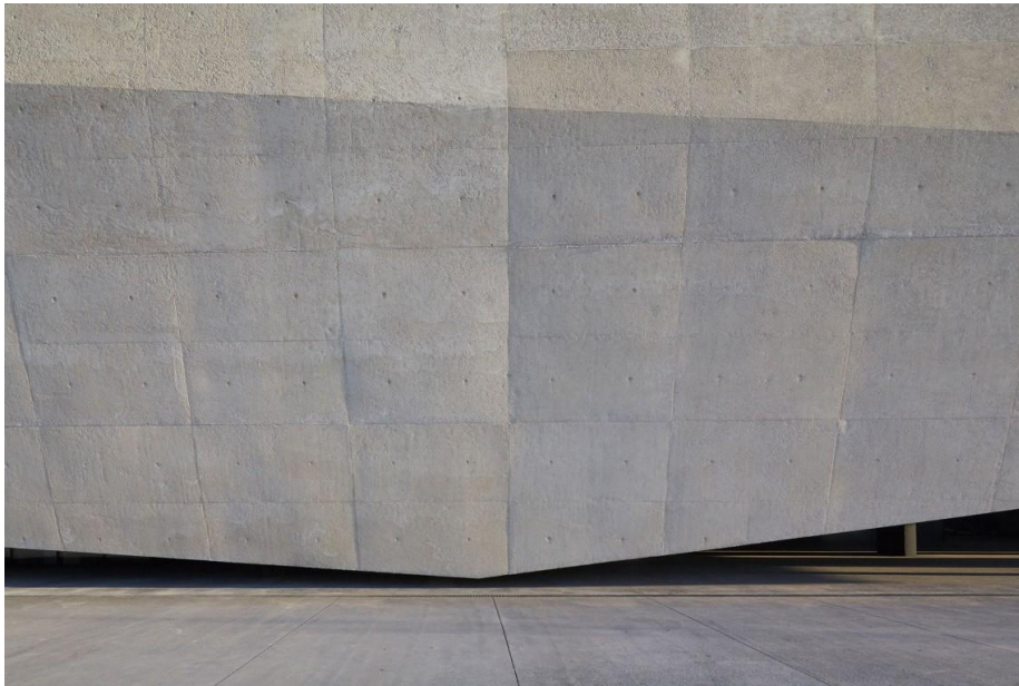
Figure 3- Lisbon Cruise Terminal (detail of one of the walls where the mixture of cement and cork was used) (Burmester, 2018)
