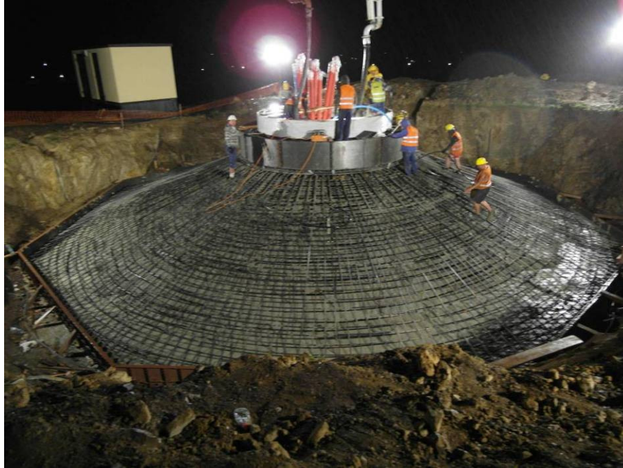
5. Concreting at night with use of halogen lamps.
