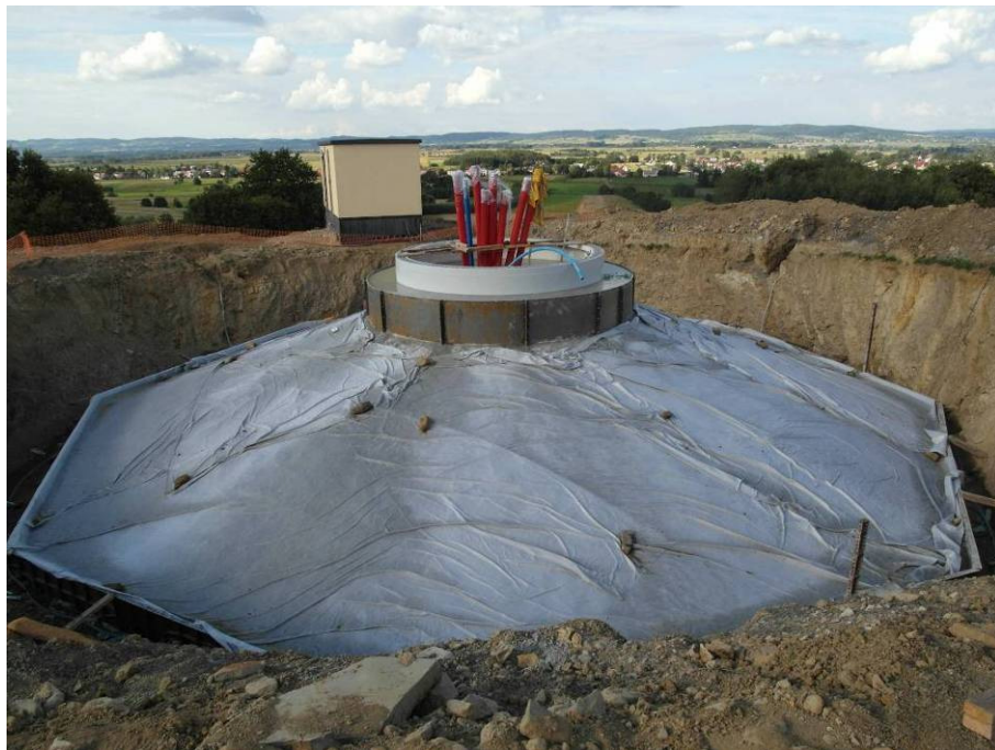
8. Curing of concrete.
