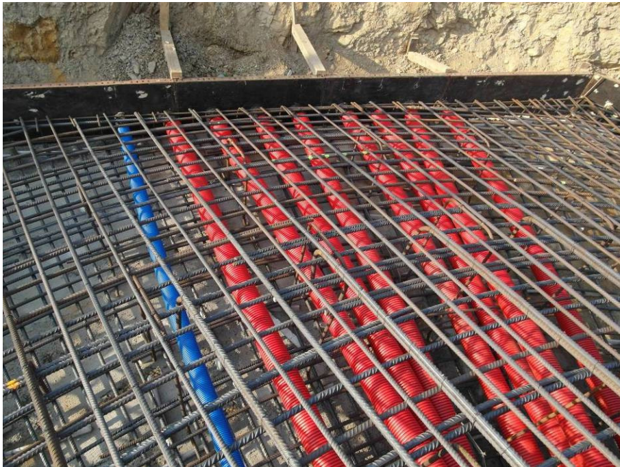
2. Cable duct pipes installed.
