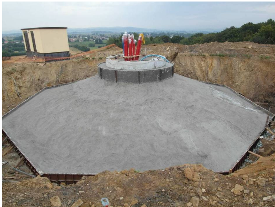
6. Foundation after concreting.
