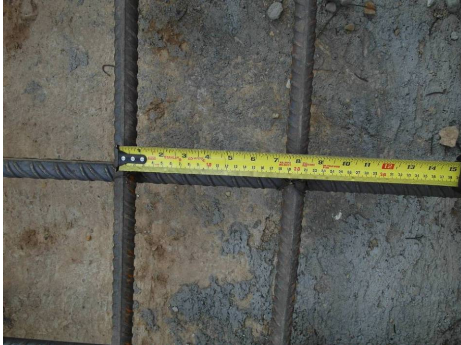
3. Reinforcement bars distance check.
