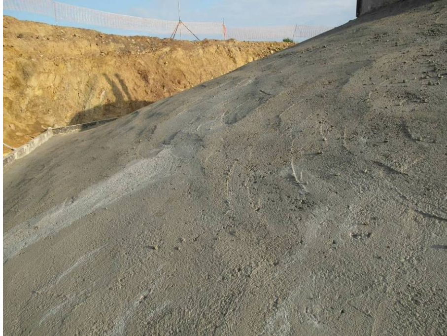
7. Trowelled concrete surface.
