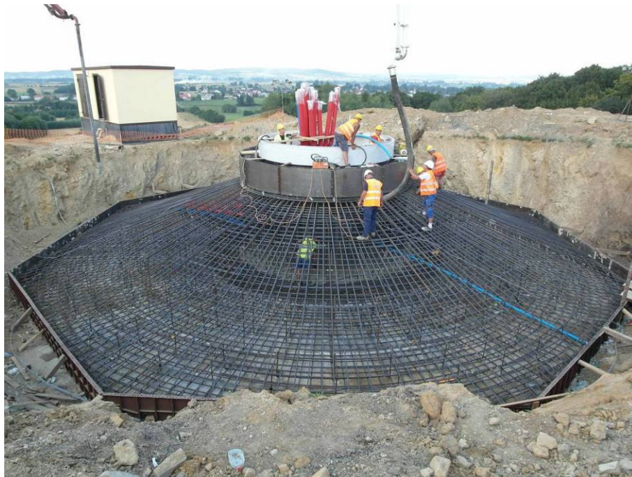
4. Beginning of concreting.
