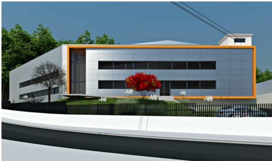
Figure 2.1: AMF plant in Guimarães.
