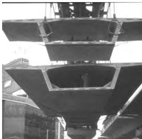
Figura 62 - Bangkok Second Stage Expressway
