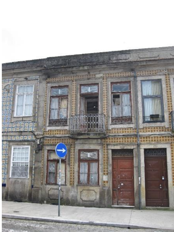
a) Fachada principal
