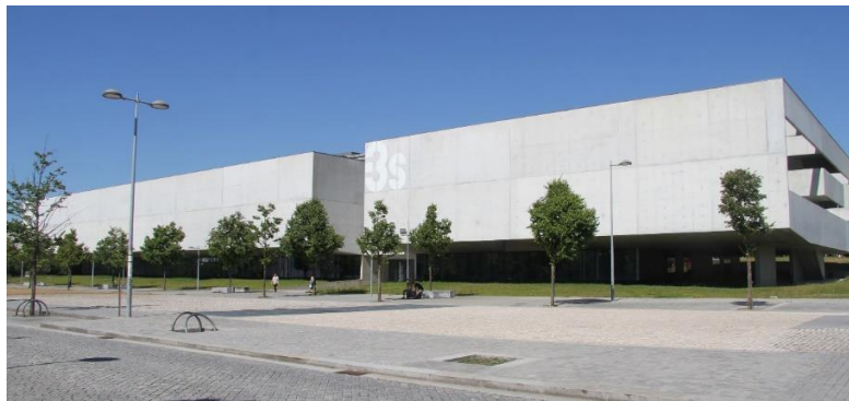
Figure 2 – I3S Building, Street view (i3s, 2024).
