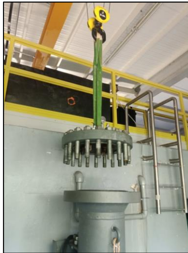
Figure 72. Pressure chamber lid being lifted with a crane
